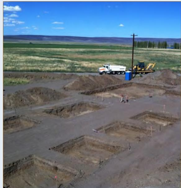
Above, beginning construction of the foundations for the power plant and cooling towers for Surprise Valley's geothermal plant near Paisley, Oregon.
